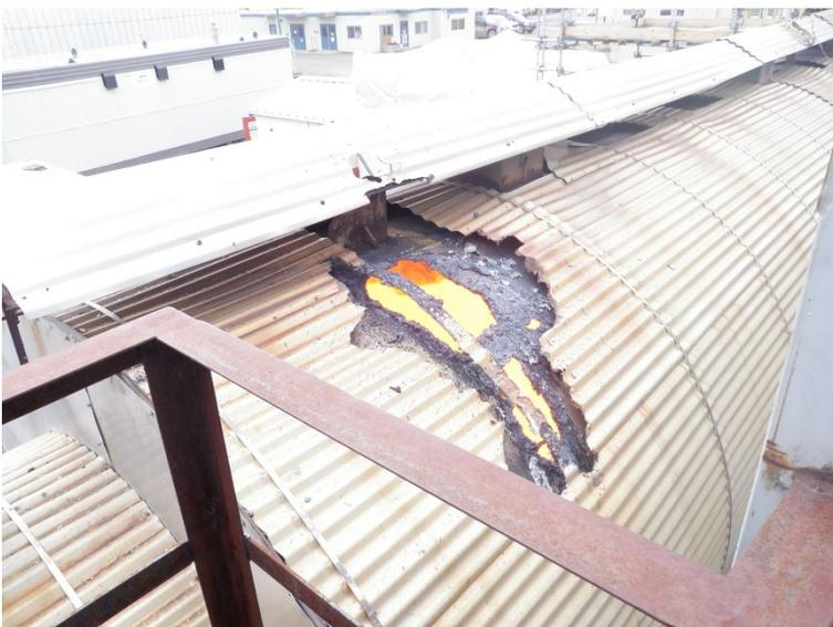
**Figure 4. Damaged shell after refractory failure**
