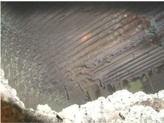
Figure 12. Damaged reheater tubes
