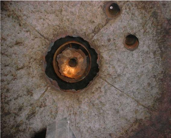
**Figure 1. Burner throat showing backfiring**
