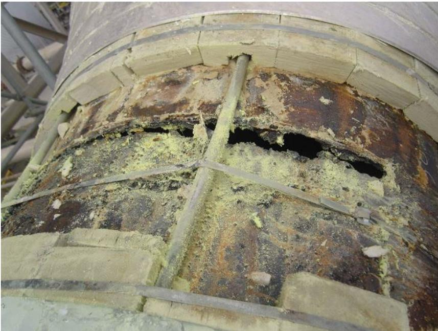
**Figure 9. Corrosion of SUPERCLAUS® bypass line**
