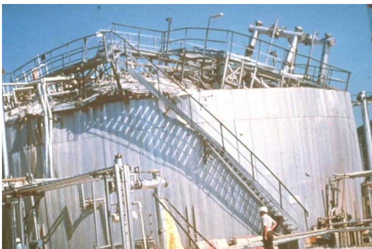
Figure 1. Destruction of sulphur tank at Greek refinery in the 1980s
